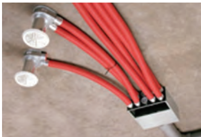
From a suspended ceiling
