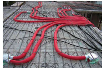
In the concrete screed
