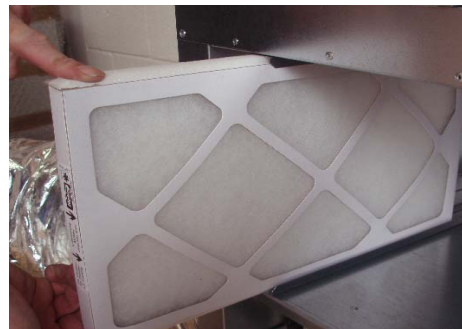
Pre-filter which protects the plate heat exchanger and the pollen filter
